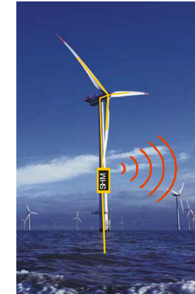
Structure health monitoring
