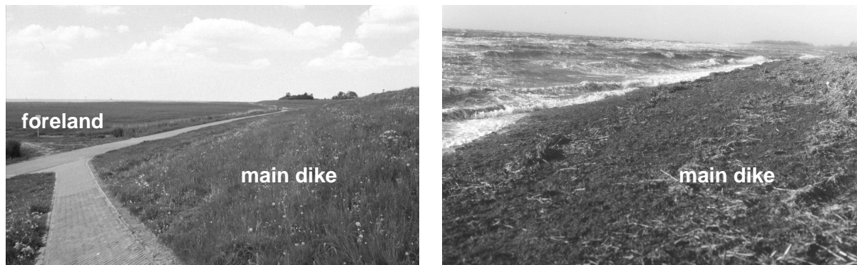
Fig. 1: Natural Forelands under Mean Tidal Conditions (left) and during Storm Tides (right)
